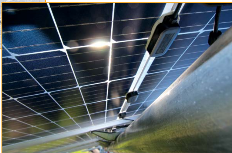
HALF-CUT CELLS The bifacial modules that Nextacker and PVEL used as the basis of this comparison, summarized in Table 1 (p. 4), have half-cut cells and mid-module junction boxes. Whereas the module backsheet material at the Nextacker site is transparent with a white grid between cells, the backsheet material at the PVEL site is fully transparent.
