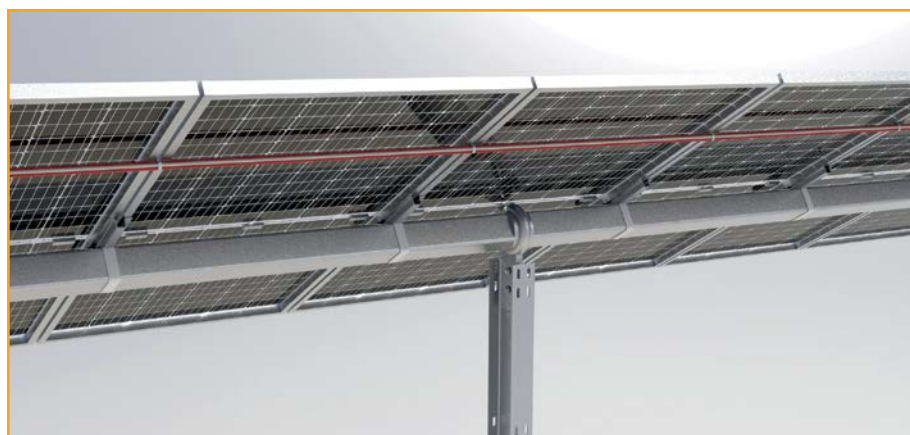
FIGURE D2 In a “super row” scenario, where DC homeruns are aggregated across multiple tracker tables, DC wire bundles are roughly two inches in diameter. The additional back-side shading in this scenario can decrease system-level specific yield by 0.25% to 0.35%.
