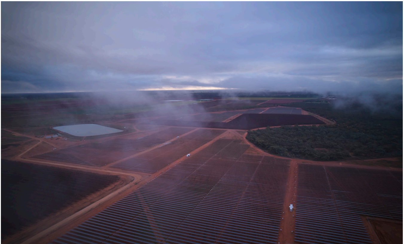
Storm over Bannerton Solar Farm, Australia
